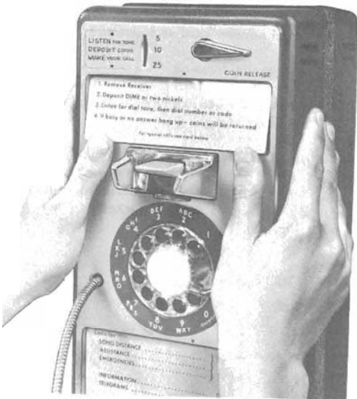
Fig. 14—Installing Instruction Cards (1C-Type)
